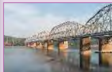
Bridge over the Yenisei River, Krasnoyarsk
